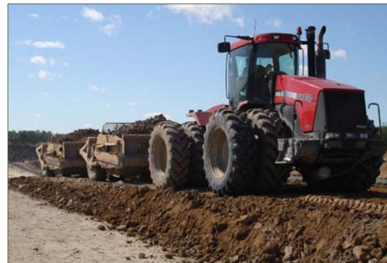
Pan scrapers have reduced compaction issues
