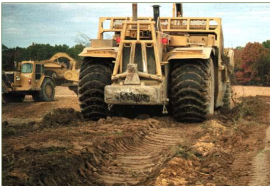
Compaction caused by twin-engine scrapers
