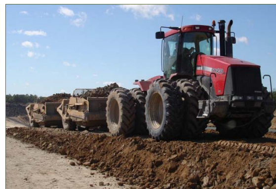
Pan scrapers have reduced compaction issues
