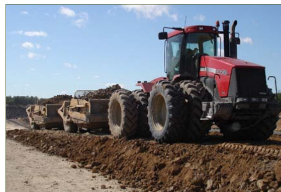
Pan scrapers have reduced compaction issues
