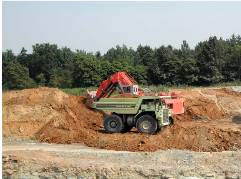
Soil loading using hydraulic excavator
